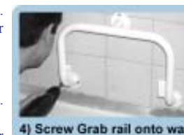
4) Screw Grab rail onto wall
