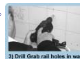
3) Drill Grab rail holes in wall
