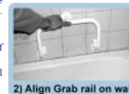
2) Align Grab rail on wall
