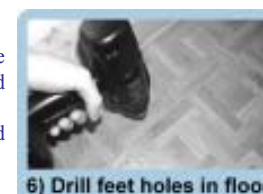
6) Drill feet holes in floor
