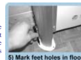
5) Mark feet holes in floor
